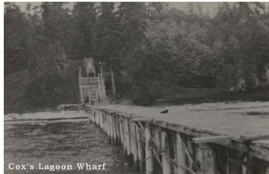
However, the 1907 Ministry of Mines report stated that a 1 1/4 mile long tramway and a 400-foot wharf with two large bunkers had been built at Cox's Lagoon, one mile south of the old wharf site. The previous site would "...not be used, because, during the stormy weather of the winter time, it offers no protection to vessels".
